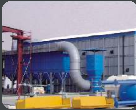
Dust Collector at site for Blast Room
